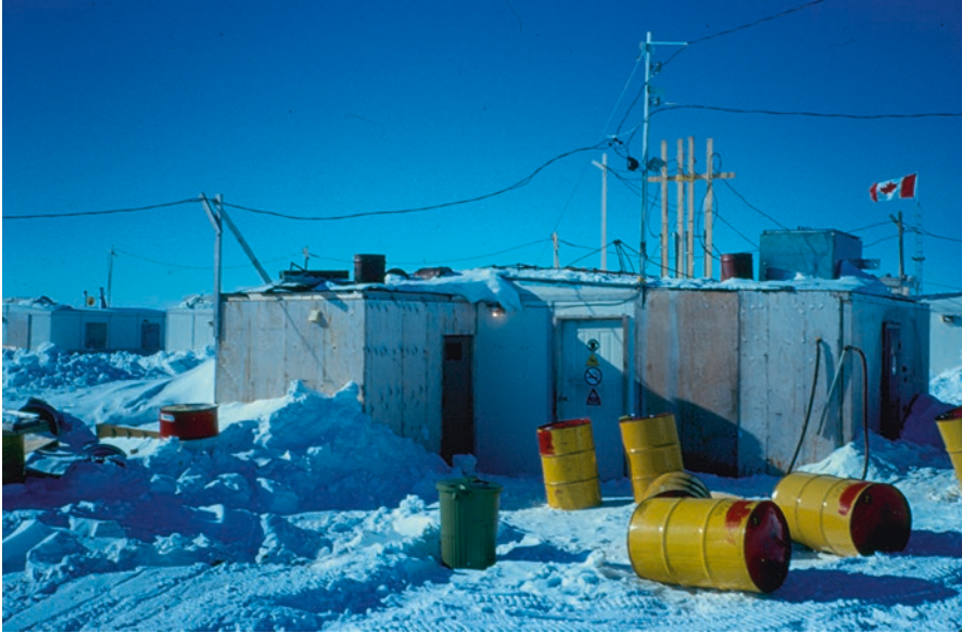
Fig. 13.4 Diesel shack for the Hobson's Choice Ice Island facility, 1990. The hut housed a 30-kilowatt generator (Source: William Althoff)
