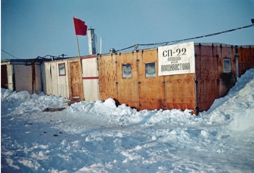
Fig. 14.7 Main complex of several interconnected prefabricated huts on drifting station NP-22 in May 1977. Developed by Russian designers Kanaki and Ovchinnikov, these comfortable mobile huts were officially termed PDKO after them, with PD standing for polyarny dom (in Russian) or polar house. The complex included mess room, kitchen, food storage, recreation room, and sauna. The sign reads: “NP-22 Vladivostok Square” after icebreaker Vladivostok , which together with M/V Captain Kondratiev delivered supplies, including the huts, for the first party of 10 in September 1973. The huts were assembled onboard before the ice camp was set up on the ice island (Photo by Igor Belkin)
