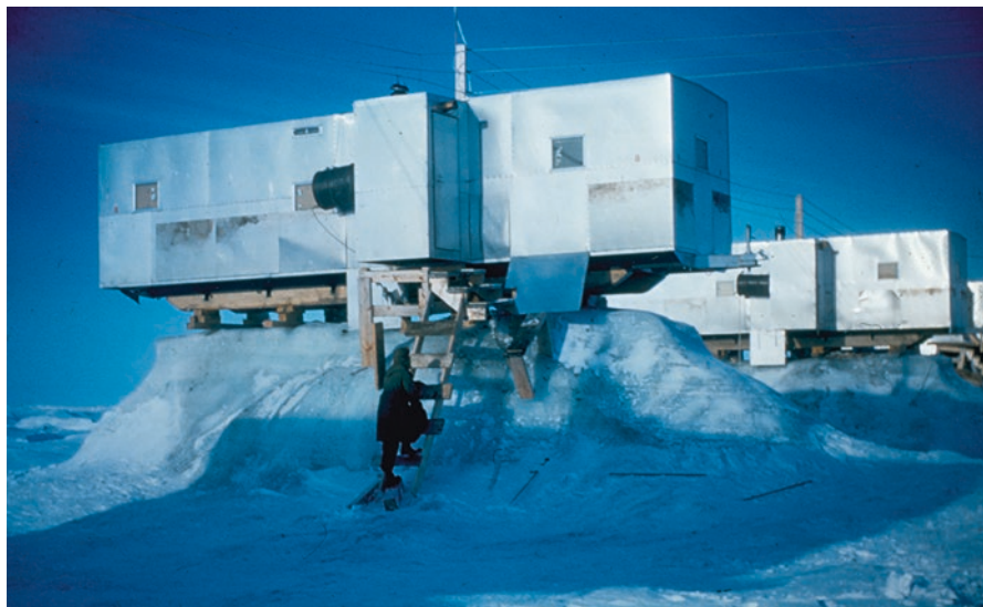
Fig. 13.7 End of the 1958 melt season: station trailers at IGY BRAVO (ice island T-3). Seasonal ablation and melt were major ice-island headaches, closing runways and pedestalling shelters due to shading of the underlying surface (Source: Dr. Gerry H. Cabaniss)
