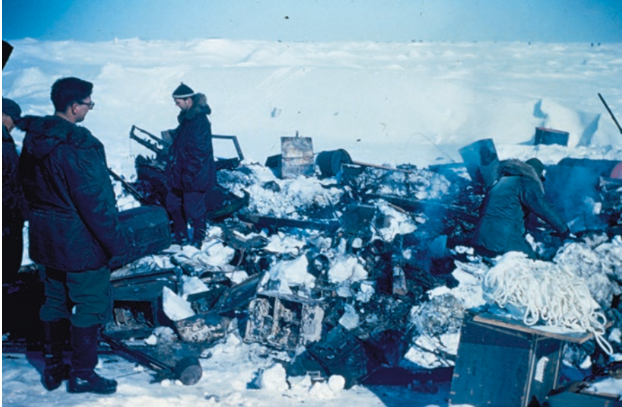
Fig. 13.6 The remains of a Jamesway shelter after a fire on ice island T-3, spring 1960. On the ice, the potential for accident and emergency haunted every camp manager (Source: Dr. Gerry H. Cabaniss)
