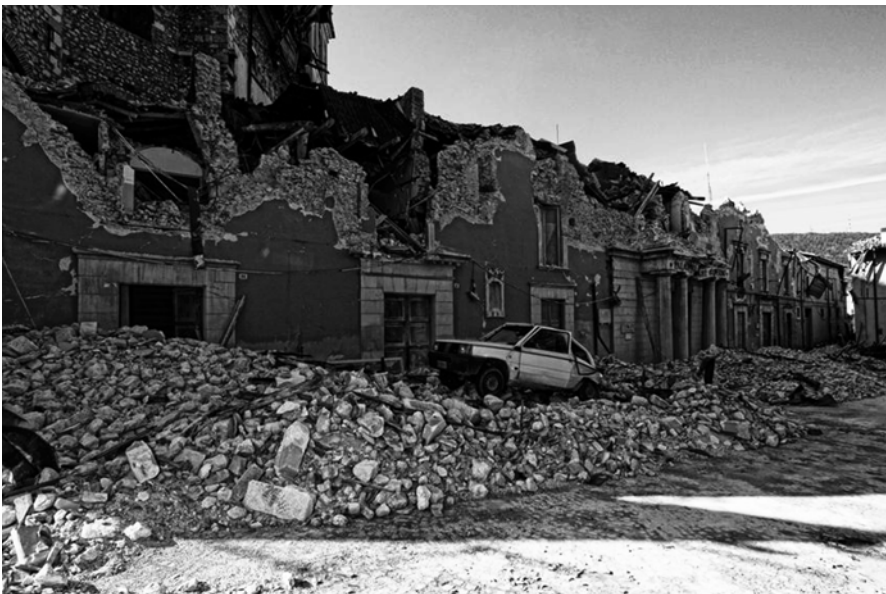
Fig. 3.6 Damage from 2009 L’Aquila Earthquake (Website of the Italian Civil Protection Department – Presidency of the Council of Ministers, http://www.protezionecivile.gov.it/jcms/en/descrizione_sismico.wp?sessionId=6EED29F25DA52C422634EE009FC67CAE?pagtab=3 )
