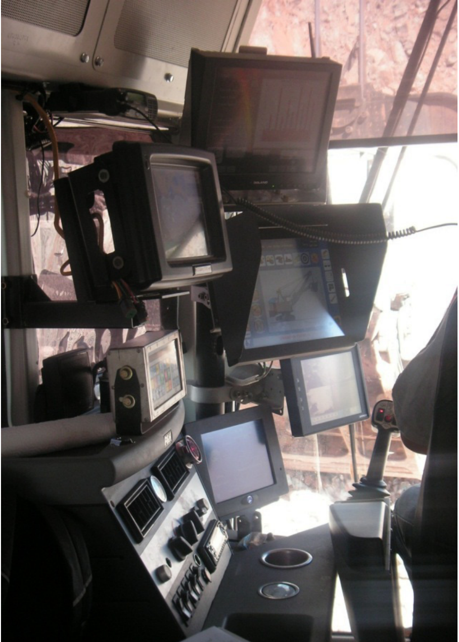
Fig. 3. Example of a technology-centric design in an electric shovel cab. Six computer monitors, communication systems, mechanical shovel controls, and a control panel clutter the cab. Clearly, this is not a user-centric design.
