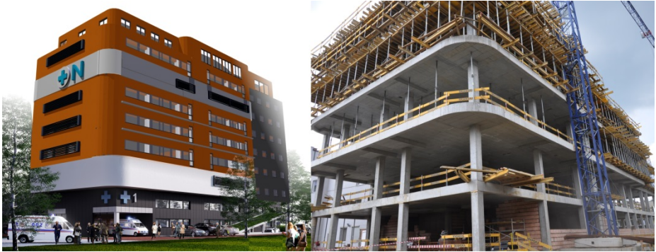
Fig. 3. Hospital in Siemianowice (Poland) under construction, 2013/2014. Photo: K. Fross 2013
