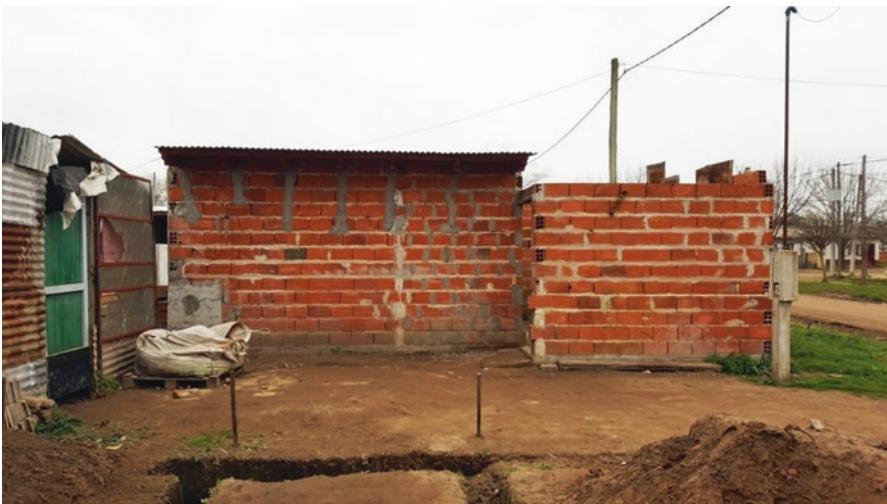
Fig. 6.15 Barrios Unidos: informally-constructed, self-built home. (Reproduced from Vexina Wilkinson 2017)
