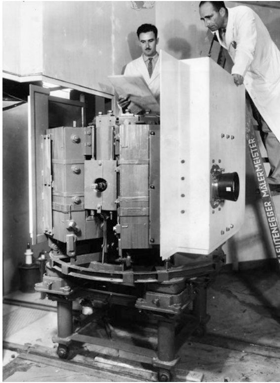
The first medical betatron was a machine for the hospital in Zurich. On the left: D. Gamper. ( Photo ABB Archives )
