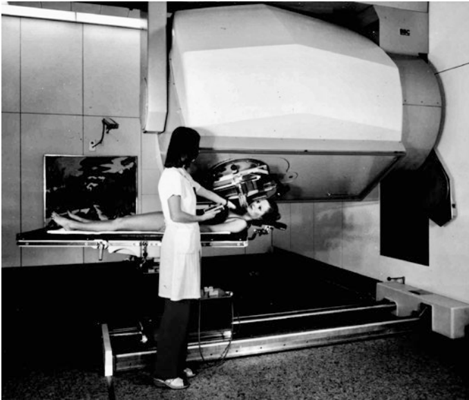
The Inselspital University Hospital in Berne in 1952 got their first medical betatron, number three in the series of 31 MeV machines. (Photo ABB Archives)
