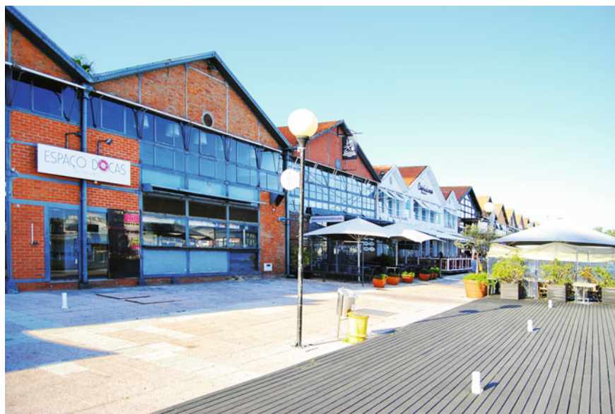
Fig. 4 Former port warehouses refurbished to host bars and restaurants in the docks of Sto. Amaro. Author: José M. P. Sánchez; released under a Creative Commons Attribution-NonCommercial-NoDerivatives 4.0 International License
