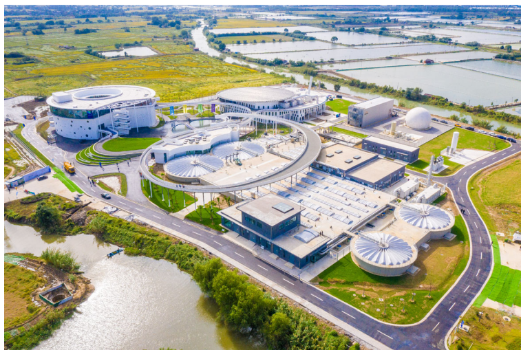
Fig. 1 The aerial view of Yixing Concept Wastewater Resource Recovery Factory.
